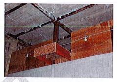
closed riser requirements. There are no separate guardrails or safety devices at the storage platform or at the open portion of the mezzanine. The short run of interior stairs between the shop area and the restroom/office level is also dimensionally non-conforming and lacks compliant handrails. OSHA regulations may also apply to these and other building elements but have not been specifically identified here.
